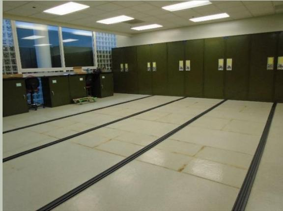
After the floor was cleared, tracks were cemented in place to allow mobility of the carriages.
