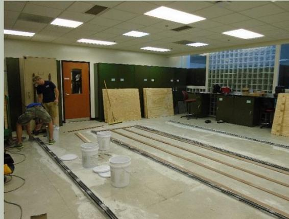
Next, an elevated platform was built along the tracks, and steel carriages installed.
