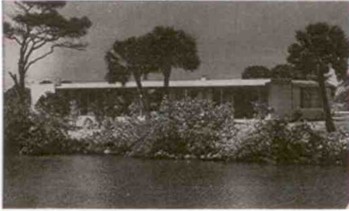
Forecast of home of tomorrow? This house was built in few days by pouring concrete into standard forms.
