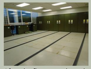
After the floor was cleared, tracks were cemented in place to allow mobility of the carriages.
